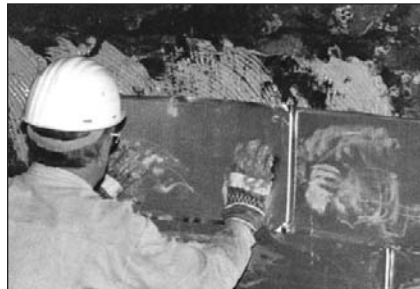
4. Press Excelfrax 1800 Flexliner into place.
