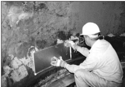
2. Place Excelfrax 1800 Flexliner over the adhesive.
