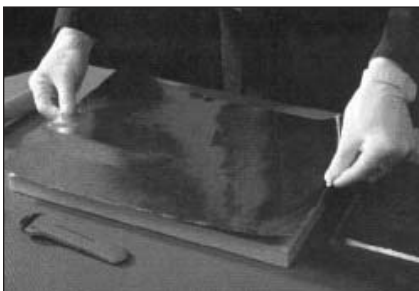
6. Cut aluminum foil to size, apply sodium silicate to foil and place aluminum foil on Excelfrax 1800 Board.
