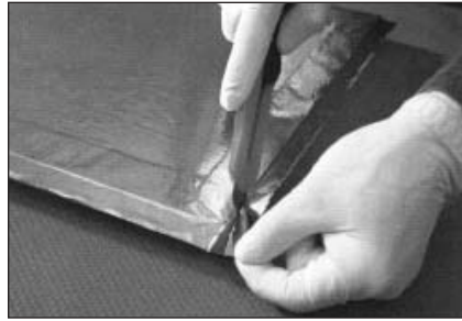
8. Trim aluminum foil with standard utility knife.
