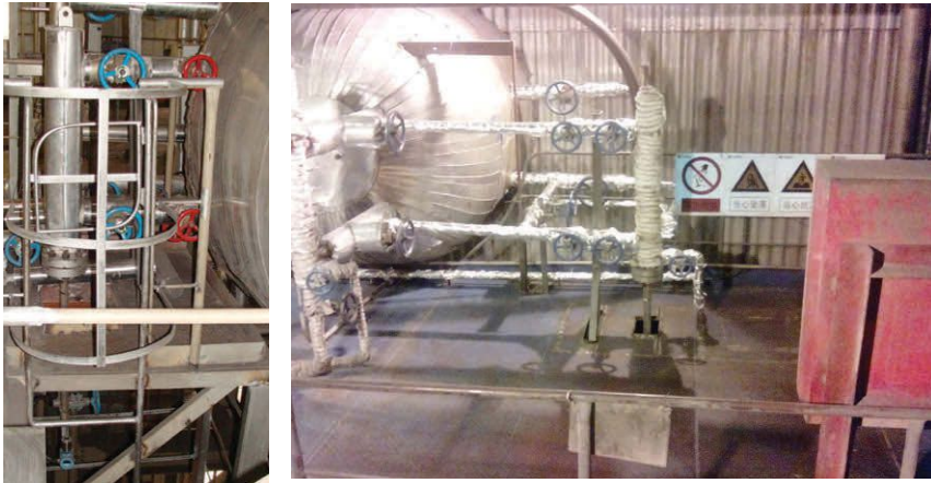
FIGURE 3 MAGNETIC LEVEL INDICATOR
