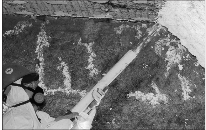
Foamfrax Installation
